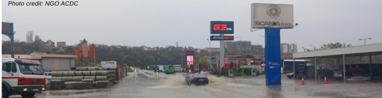
Image: 18. Nov. 2025: Entrance Mitrovica, industrial zone (former FAFOS) poor runoff management practice
